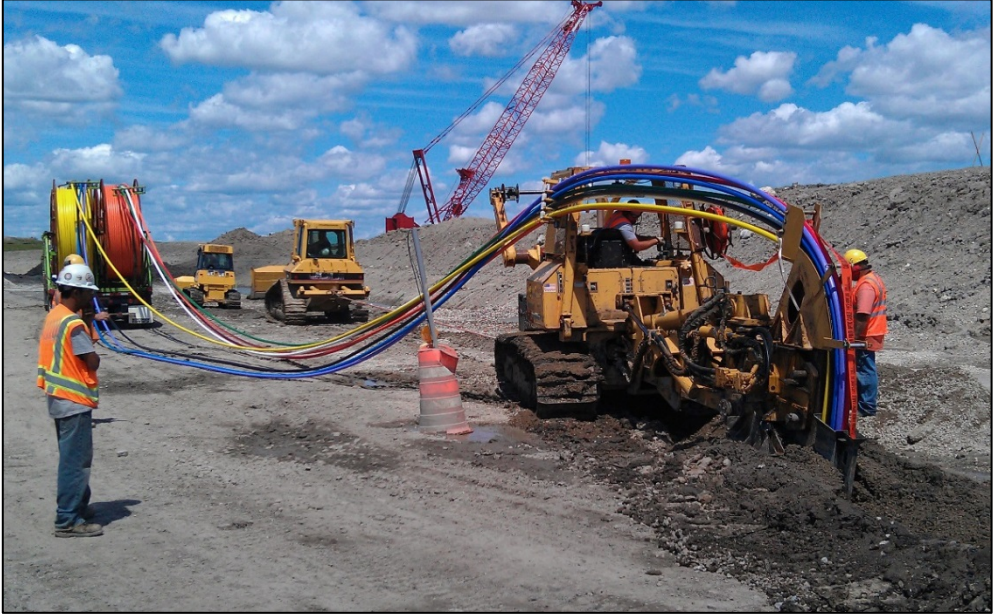
Figure 9 Example of Vibratory Plowing of Conduit
