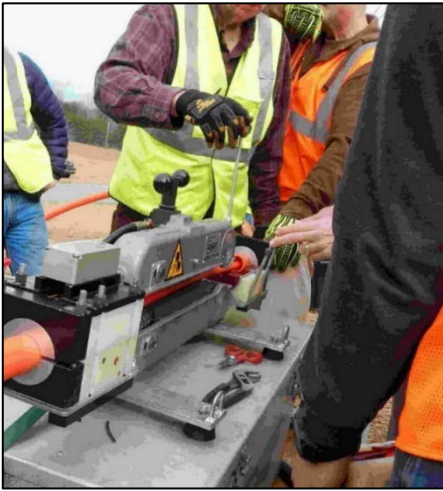
Figure 18 Jetting Microduct
